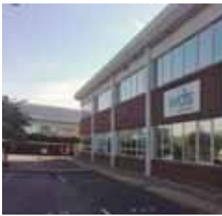
Call centre retrofit. Woodhouse Environmental Services Ltd. Bourmemouth, UK. VRF
