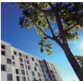
New residential building. 176 flats Xàtiva, Spain. ECO G
