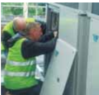
The National Grid's. Call Center refurbishment. Hinkley, UK. ECO G
