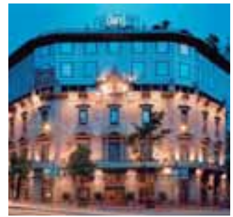
Hotel refurbishment. Hotel Claris 5 * Barcelona, Spain. ECOi
