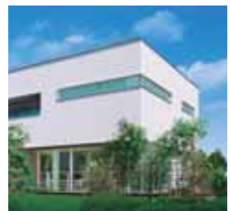
Smart House. Ariake, Tokyo. HVAC and the combination of solar power generation, fuel cells and storage batteries.
